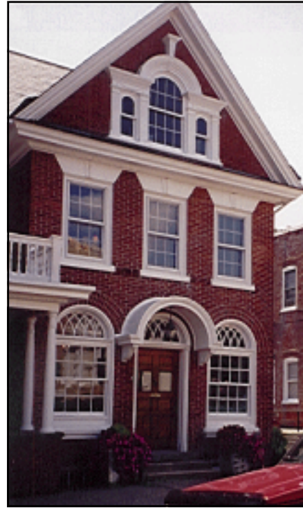
This well kept building is an excellent example of Georgian revival architecture. The brick work pointing is sound and all the exterior wood work including the windows and cornices remain and are properly painted.
